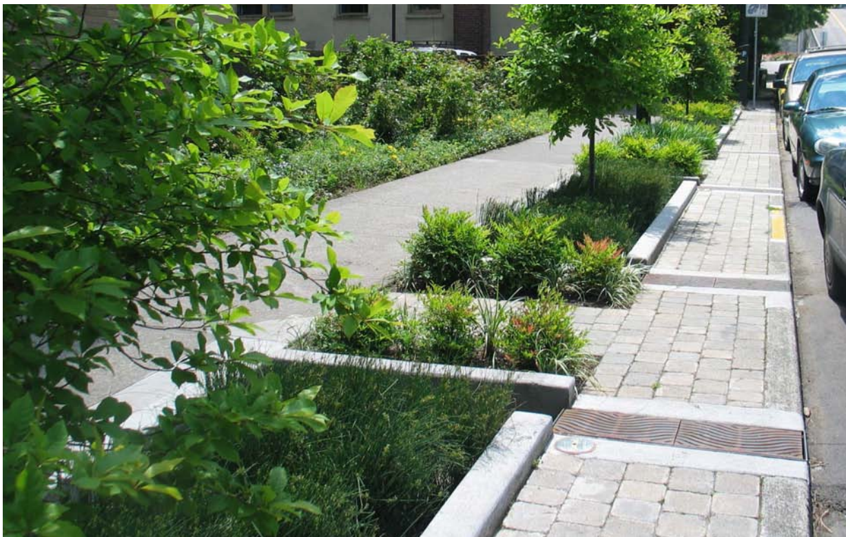
GREEN STREET WITH BIOSWALES AND FLOW-THROUGH PLANTER
